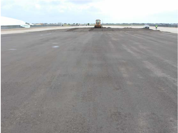
Figure 12 Bulk grain storage facility floor application
