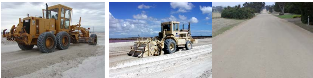
CALGRIT trials and mixing (left) unsealed sheeting (right)
