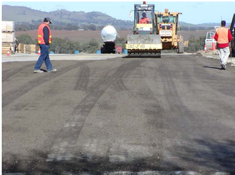
Weckert Road Tanunda (Booth Transport Access) Pavement life ESA's
