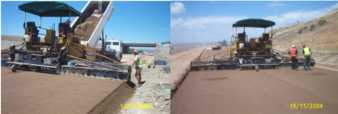
Figure 13 Paver laying CTB
