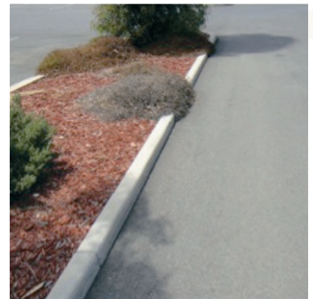
Figure 1. Bunnings completed carpark
