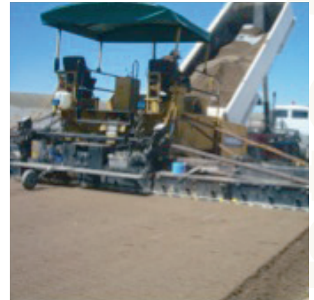
Figure 1. Aggregate paver laying CTB manufactured from recycled pavement material
