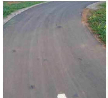
Figure 1 – popping in path surface
