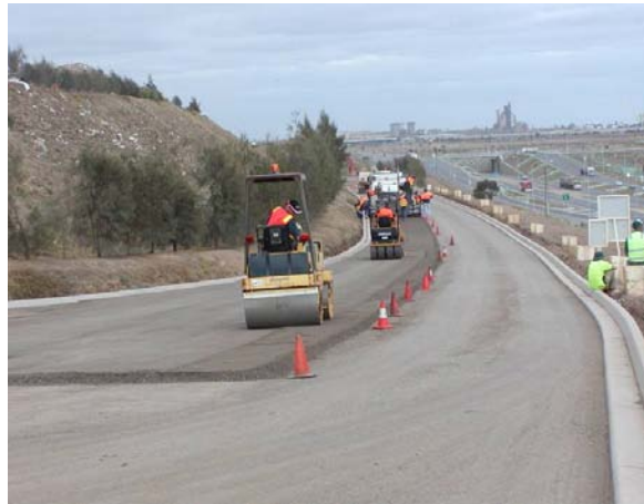
Figure 7 Wingfield – compaction
