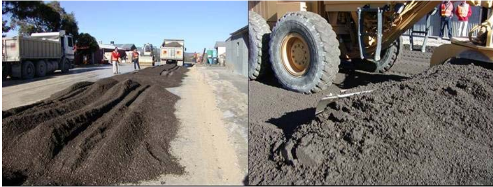
Figure 3 Tanunda – placement and grader spreading
