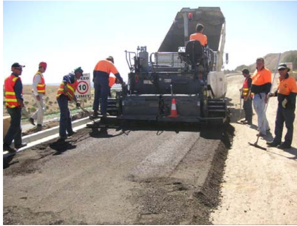
Figure 6 Wingfield – paver construction
