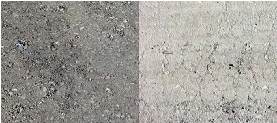
Figure 5 Tanunda surface – before and after slurring
