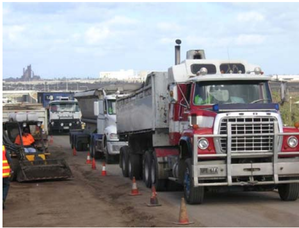
Figure 9 Wingfield – trafficking during construction
