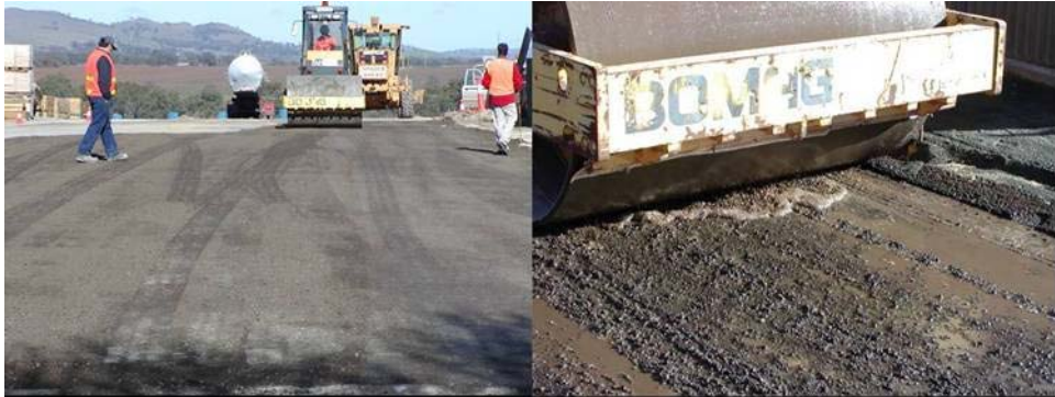
Figure 4 Tanunda – compaction and surface finishing
